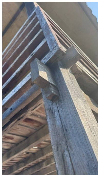
Figure 2. Unique lock system at each corner of a traditional Mandar house Source: Researcher's Processed Data, 2025
